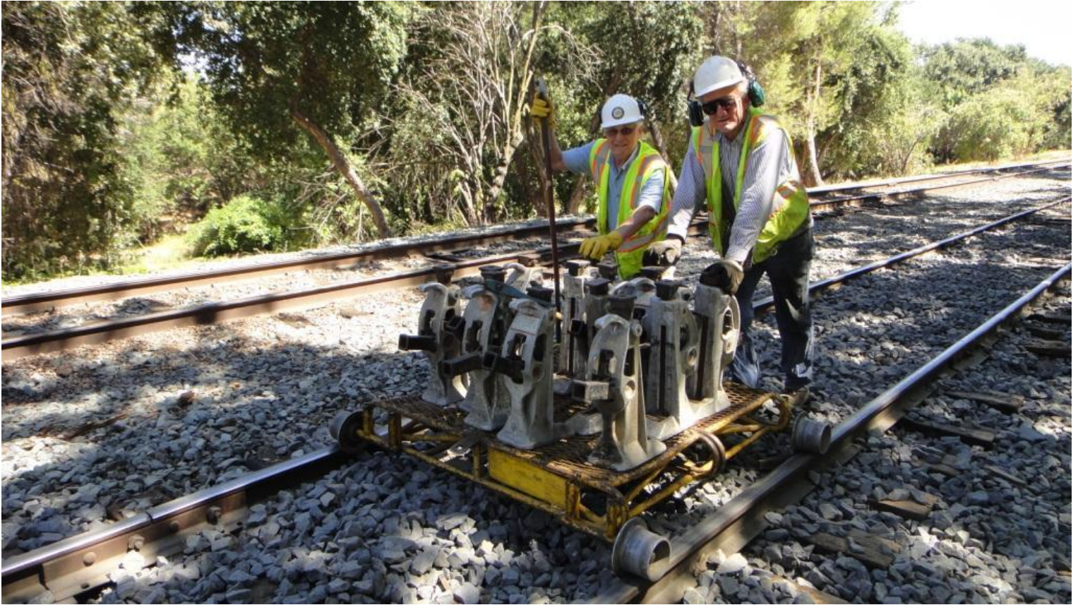
Mike W. and Steve collect the jacks on the Nolan Track Cart after a successful leveling operation
