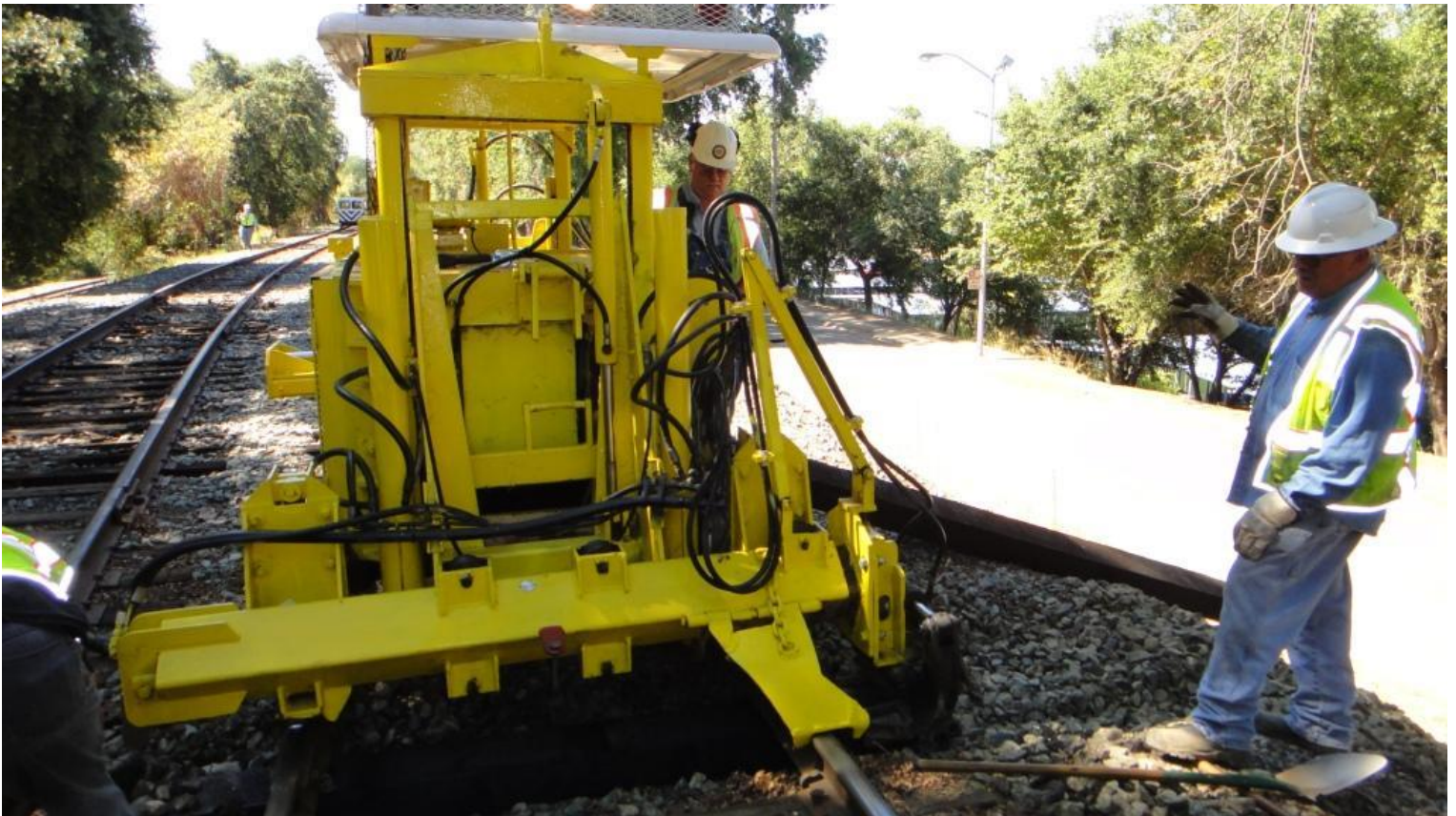
Scott guides Chris on the 125 in order to get a tie under a comp-joint properly positioned
