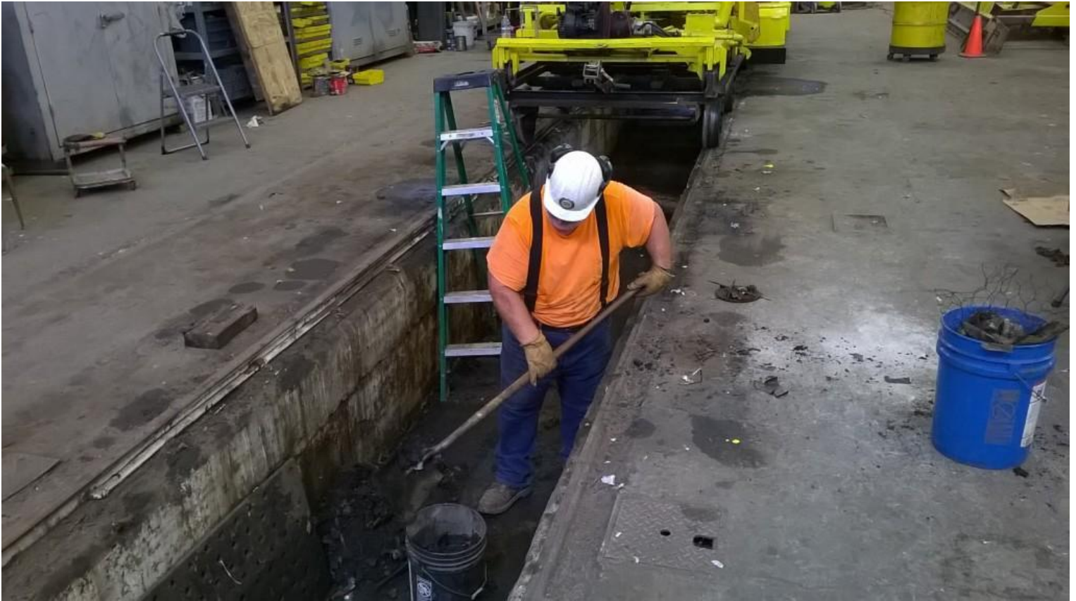
Frank shovels out the muck from the Bay 4 pit
