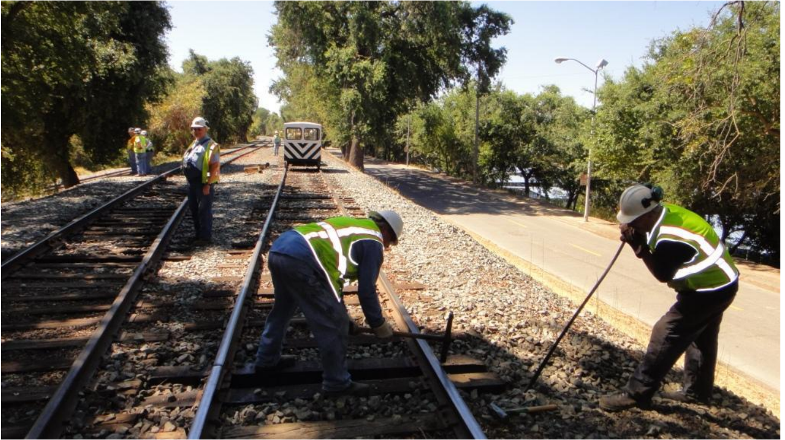
Fred nips while Scott drives spikes on ties under a comp-joint
