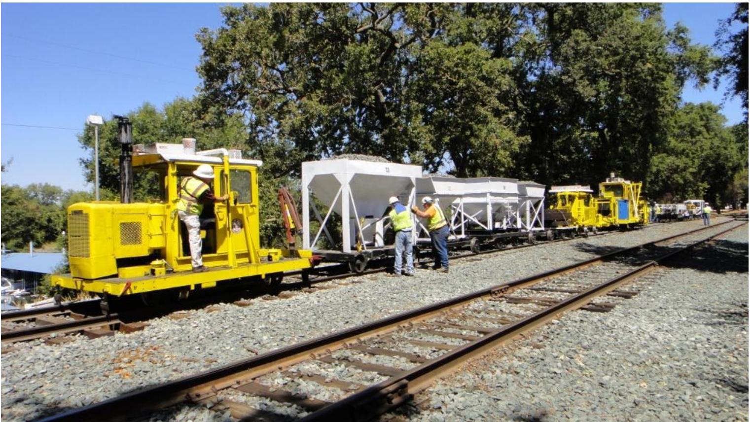
Meanwhile, Mike H. pilots the Kalamazoo tug while Mike M. and Frank W. drop rock from a ballast hopper over the "hole"
