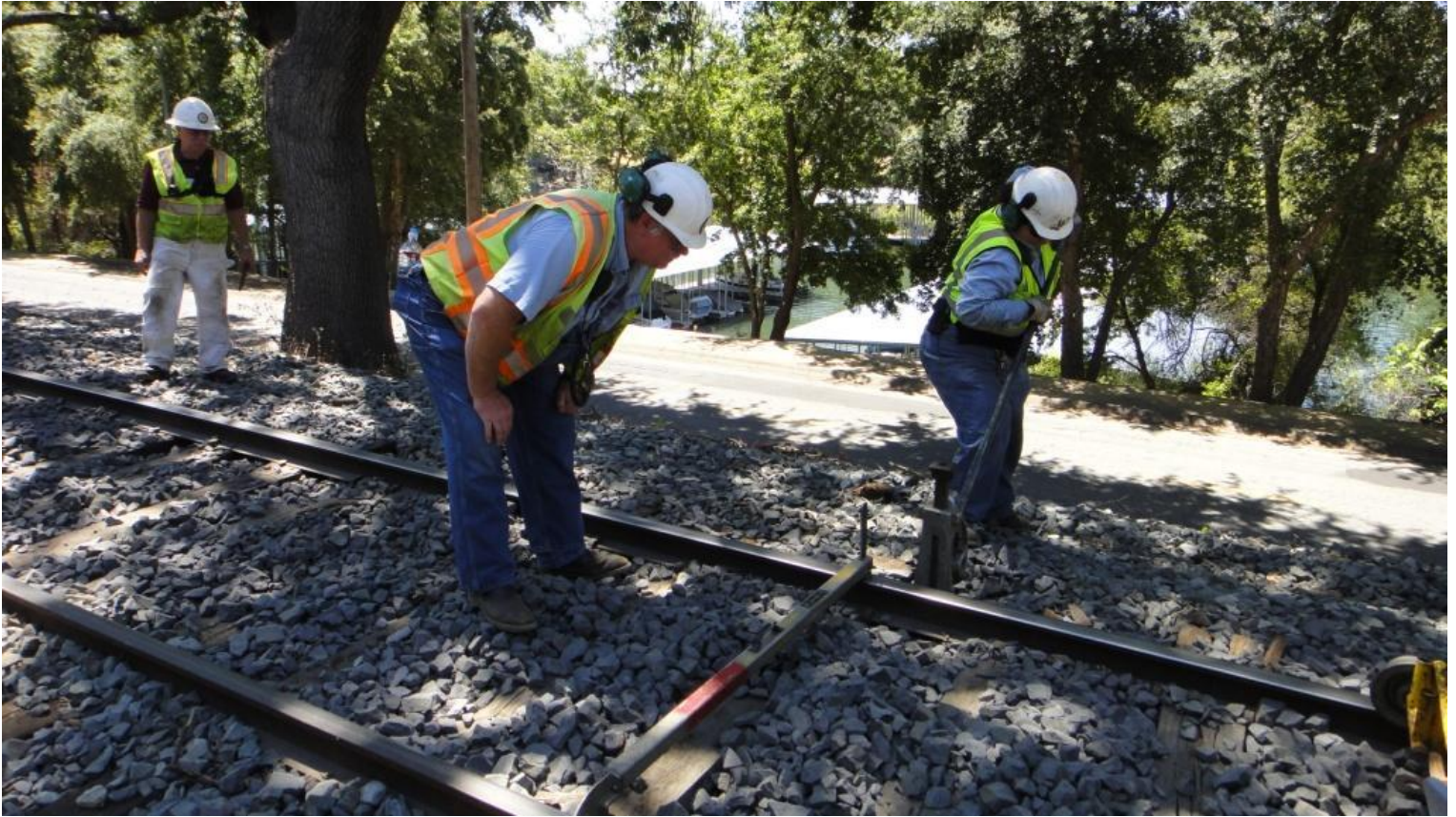
Chris keeps an eye on the level as Heather jacks-up the west rail
