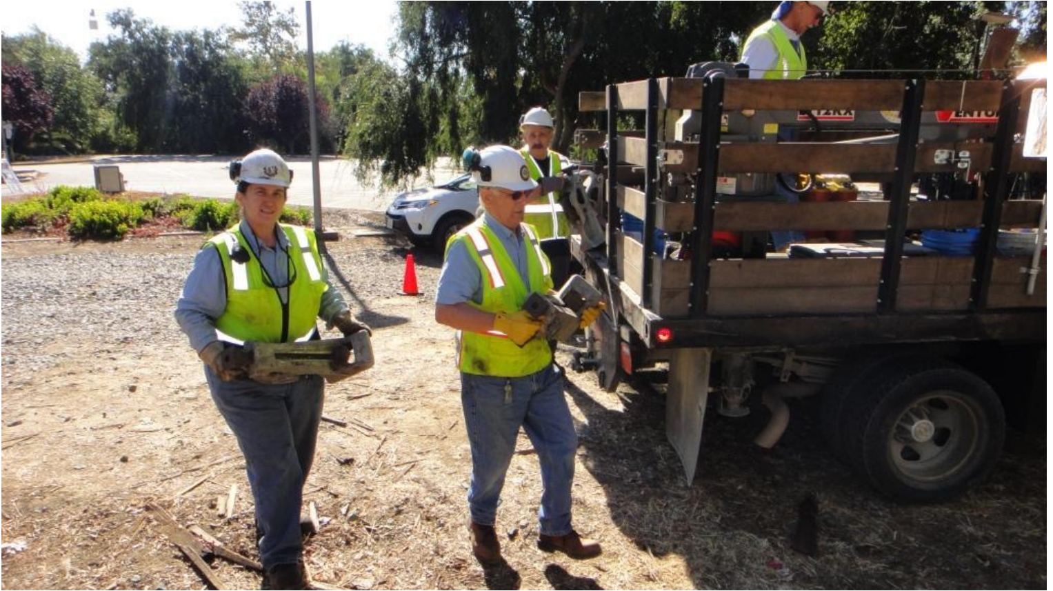
Heather and Mike W. transfer track-jacks from the truck to the work-train
