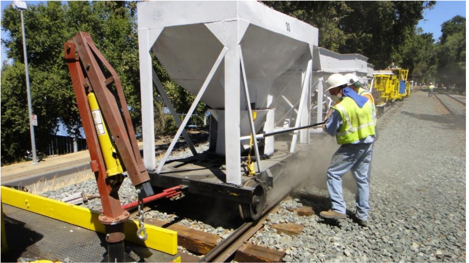
Mike M. and Frank W. dumping rock onto the line
