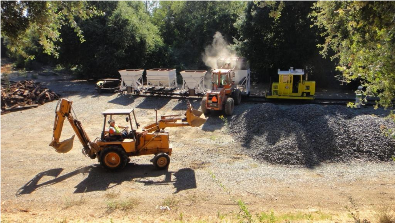
At Setzer, Iceman in the back-hoe and Frank W. in the loader fill the hoppers with rock
