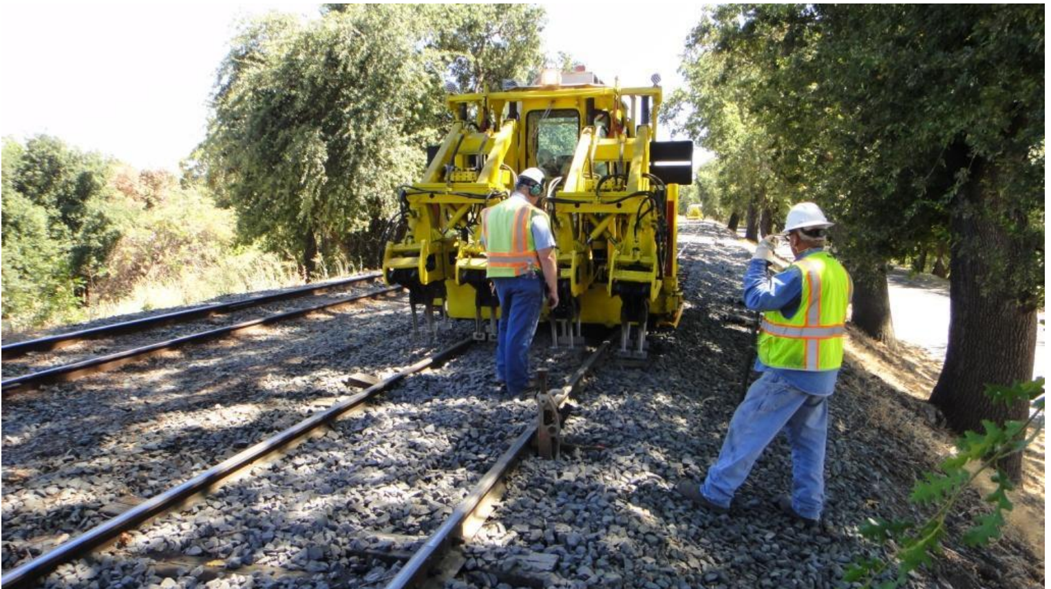
Mike H. brings in the tamper. Chris guides him and Scott prepares to pull a jack as the tamper approaches
